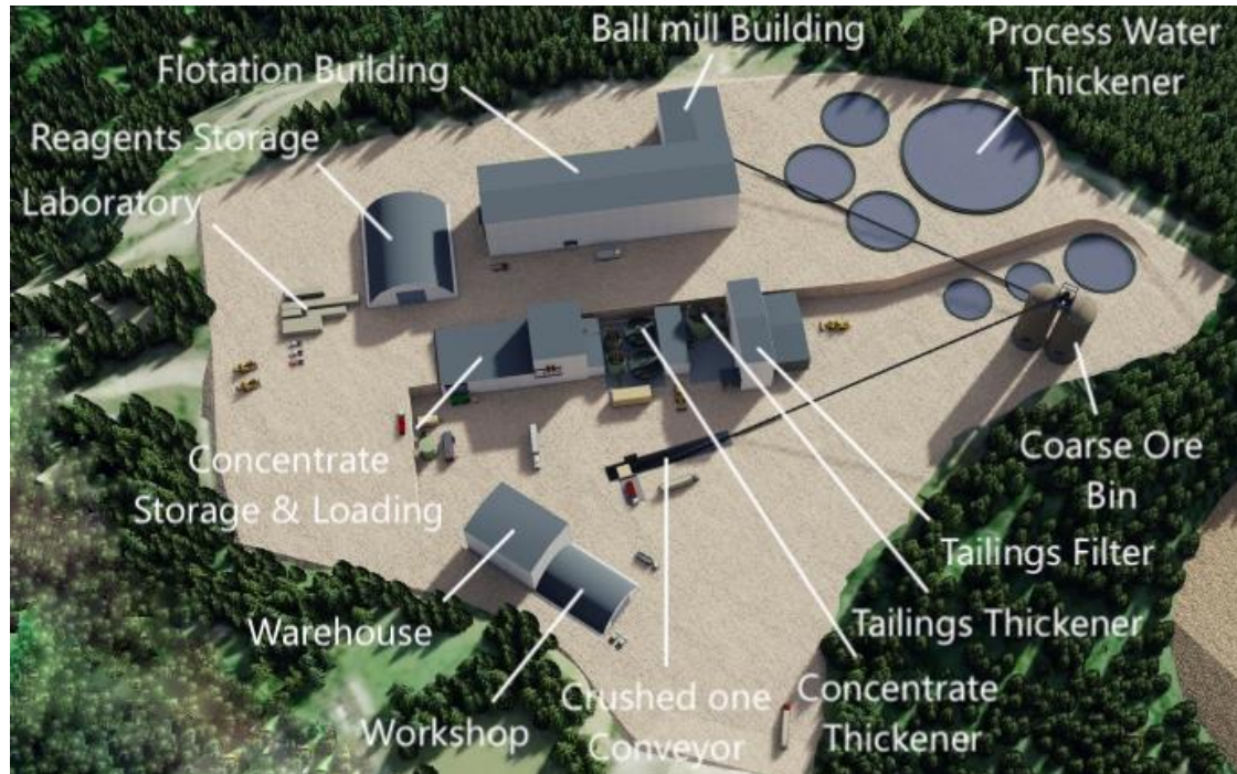
Figure 9: Isometric view of the Vares Processing Plant
