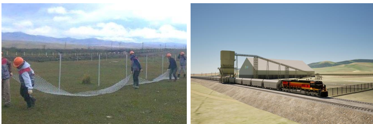
Figure 2: Fence installation around the perimeter of the 30-ha land-use permit area at the ERT site (left) and conceptual render of the ERT transloading facility (right)
