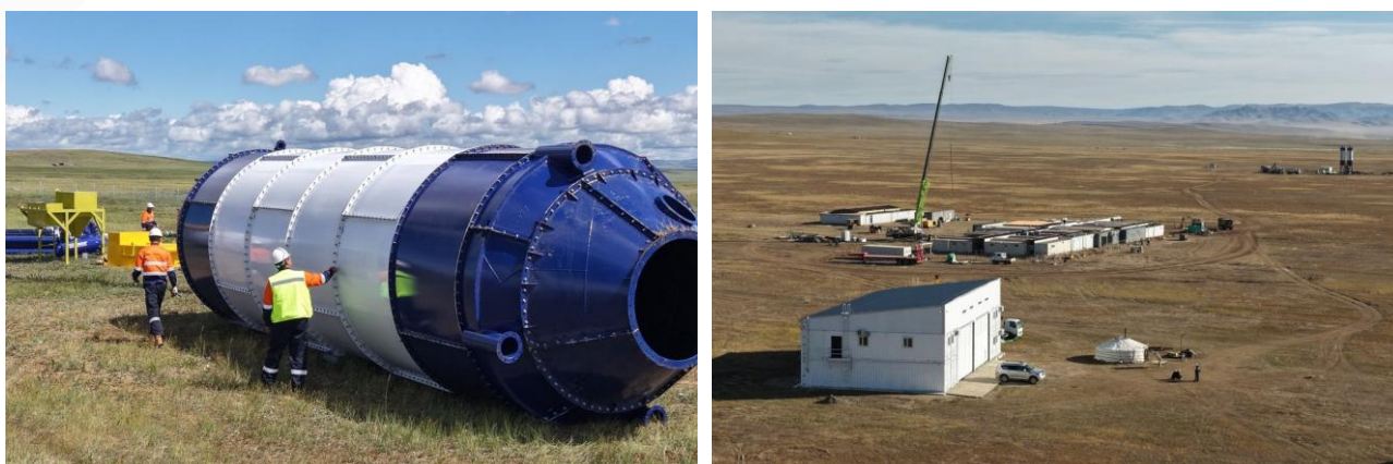
Figure 1: Subcontractor personnel inspecting concrete batching plant equipment delivery (left) and establishment of the site workshop/warehouse and contractor's accommodation (right) at the CHPP site
