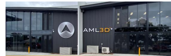
Aus Technology Centre – North Plympton
