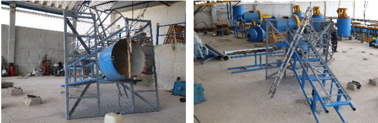
Figure 5: Cyclone tower construction
