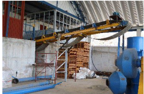
Figure 3: Mill feed conveyor installation
