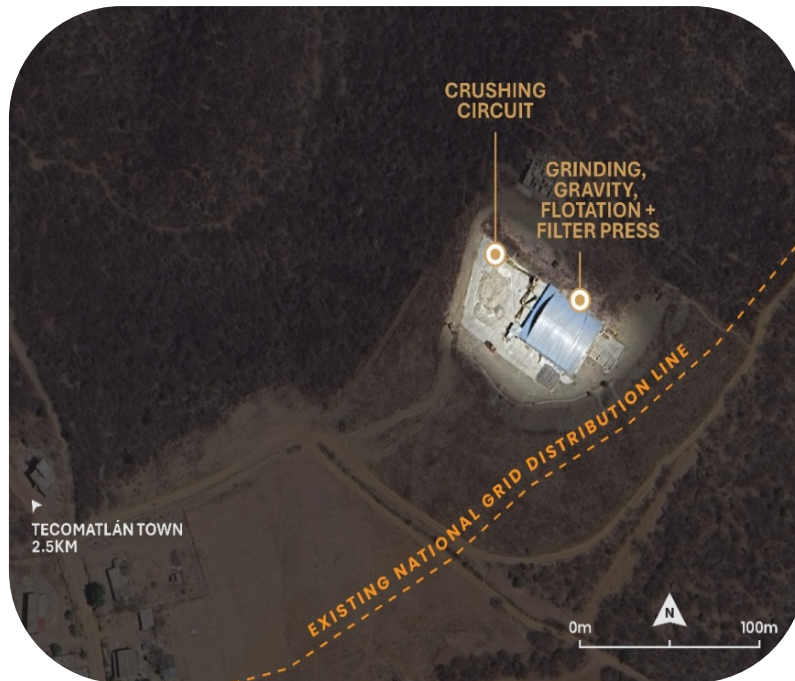
Figure 1: Below: ANT's Tecamatlán antimony processing facility in Puebla, Mexico
