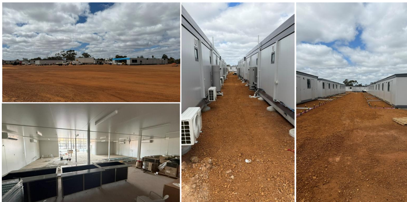
KGP Workforce Accommodation Village under construction.
