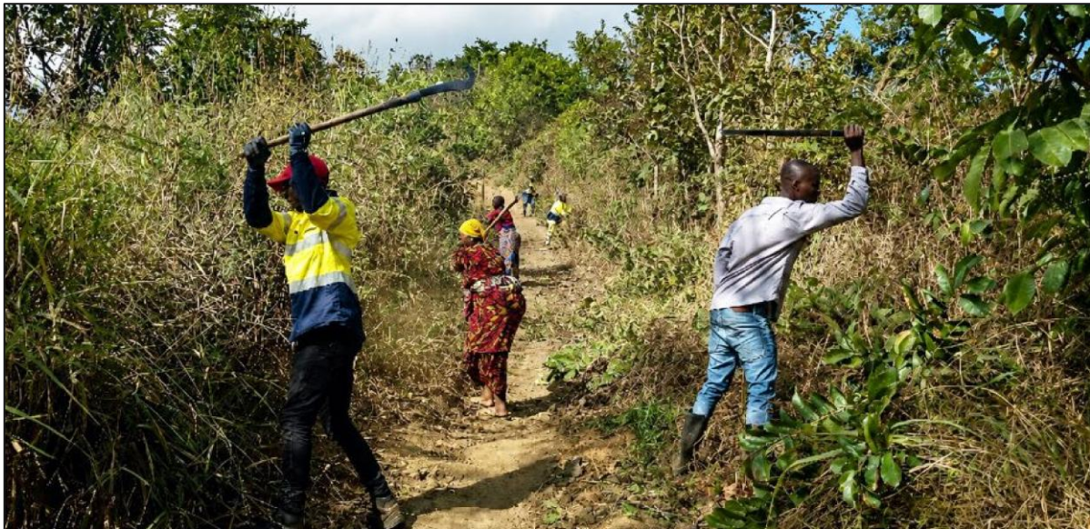
Figure 1: Kisewe Village Improving Community Access Tracks
