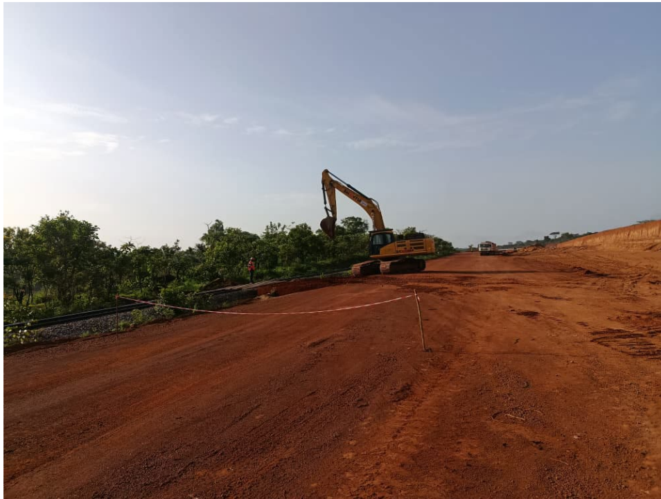
Image 2: Site works at IRF
