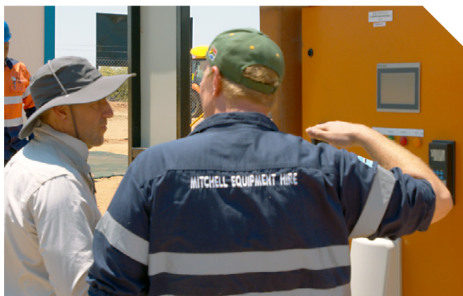
Figure 22 | SCADA operation and control system for injection pumping, Ngami.
