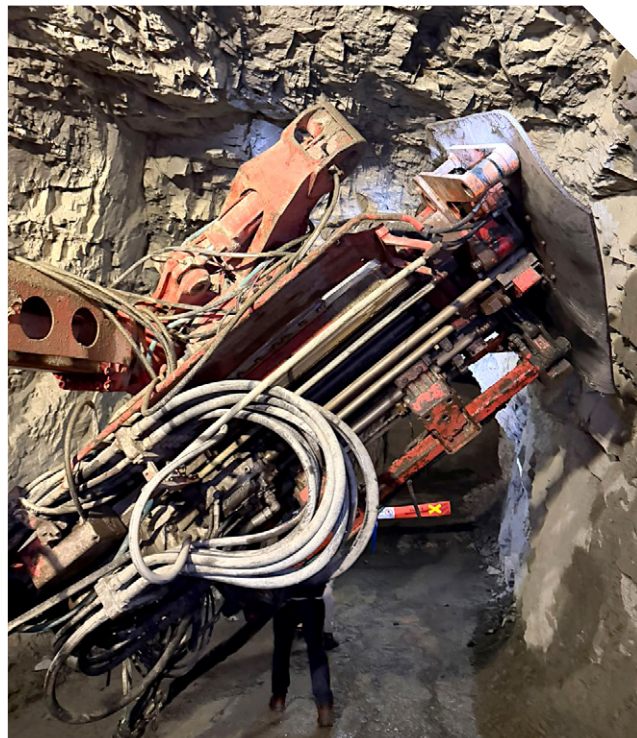
Figure 7 | Underground development at the Sierra Atacama mine
