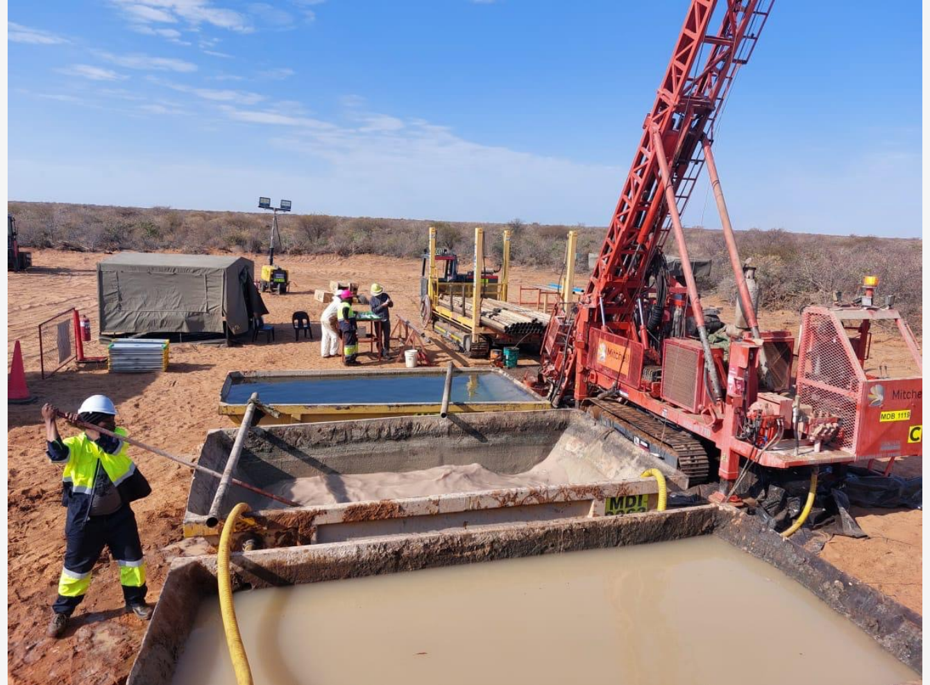
Figure: Diamond drilling at the Ngami Copper Project
