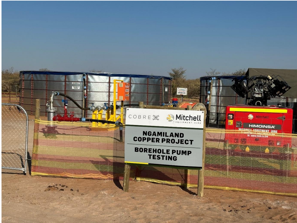
Hydrogeological pump and injection testing, NCP Botswana
