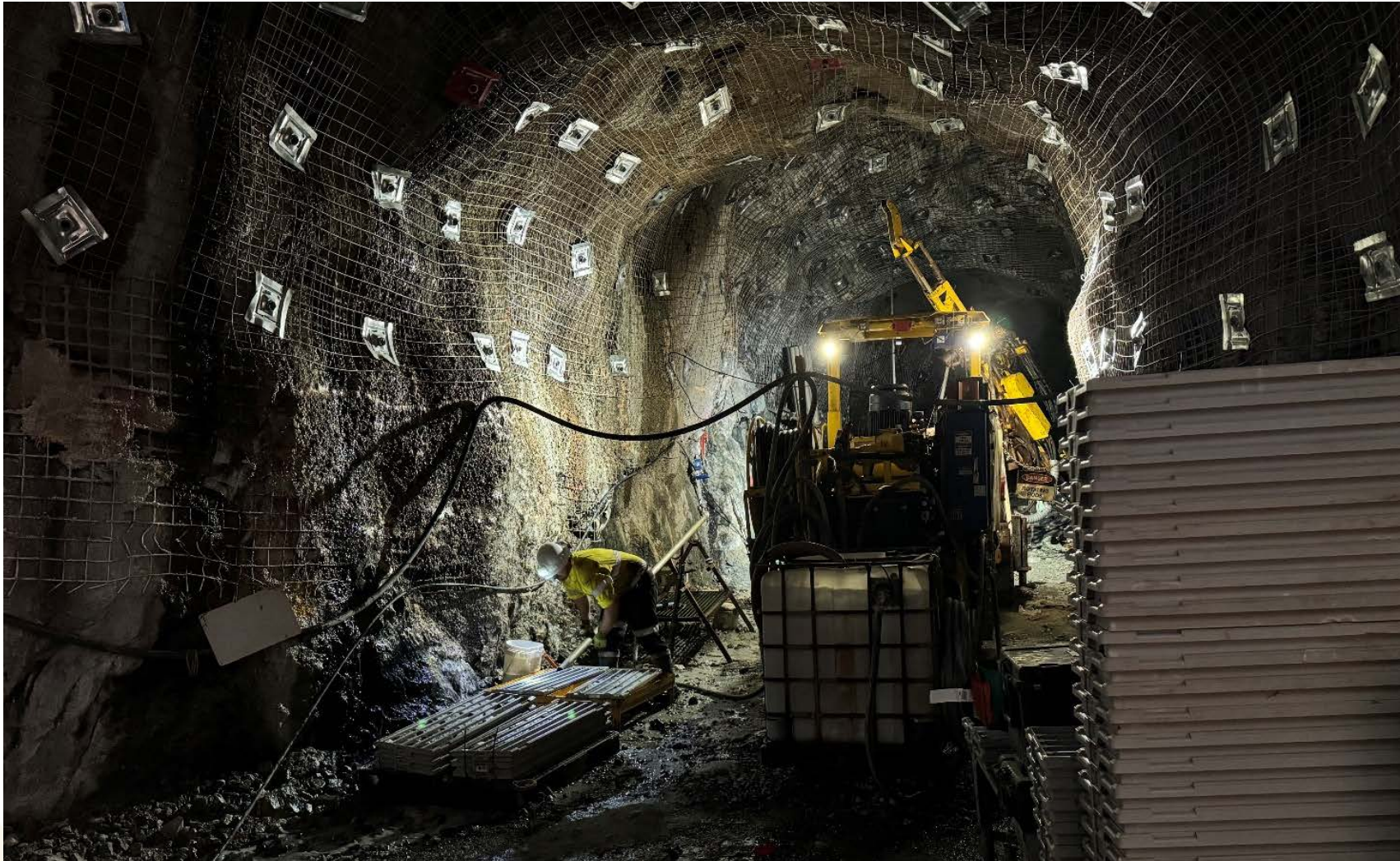
Figure 5: Rehabilitation progress and grade control drilling in the Plutonic East decline
