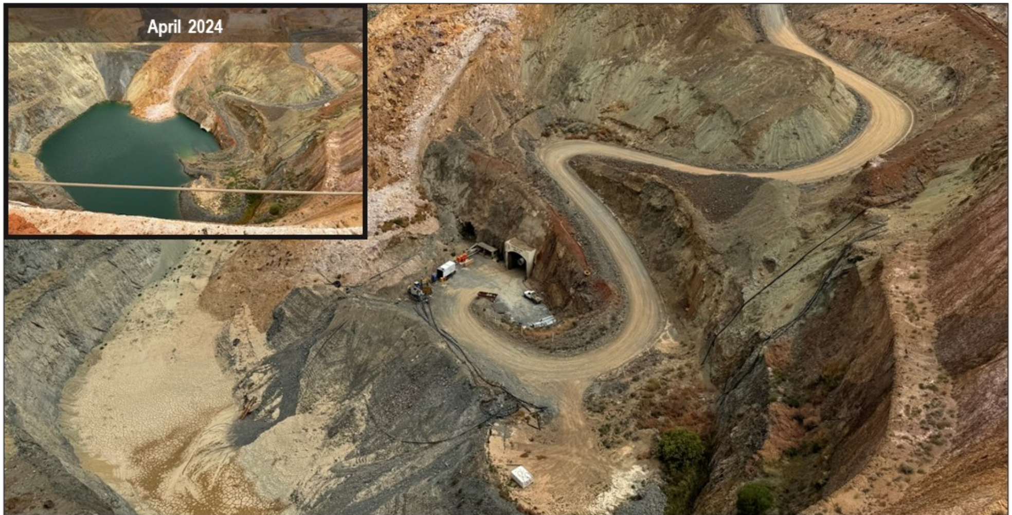
Figure 6: Dewatering progress at Plutonic East
