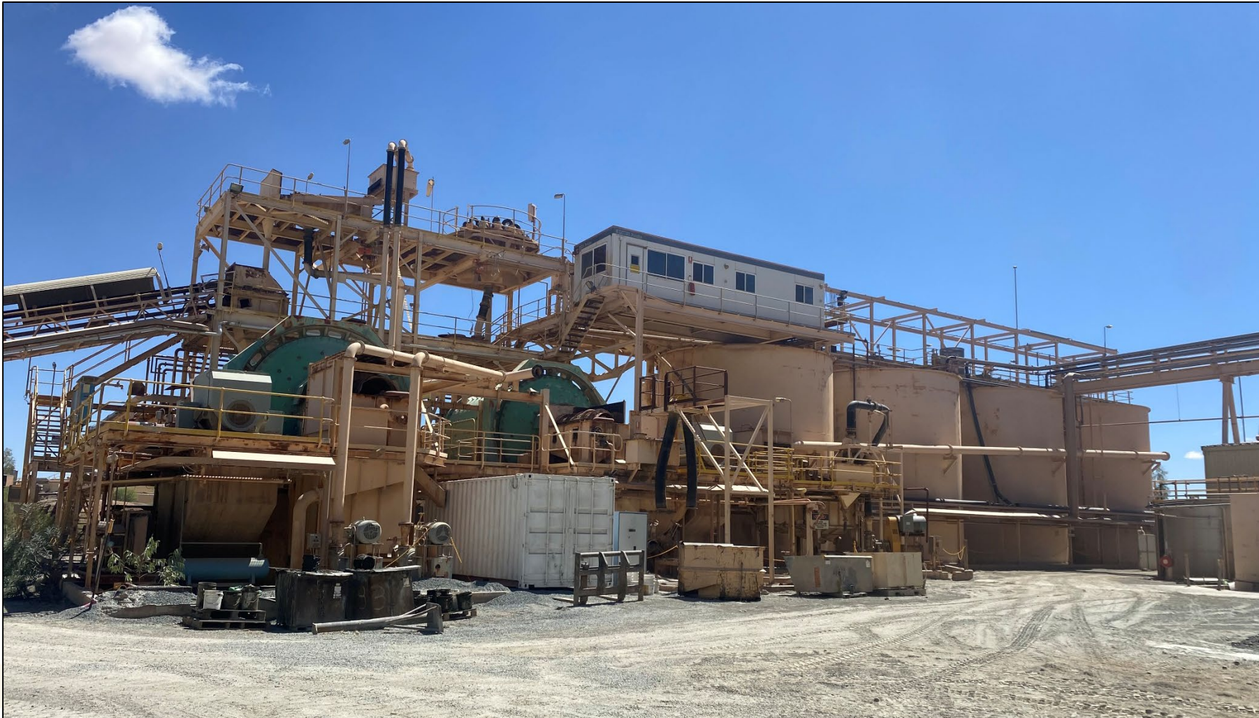
Figure 5: Plutonic processing plant 2 (PP2) showing SAG and ball mills, leach tanks and adsorption tanks
