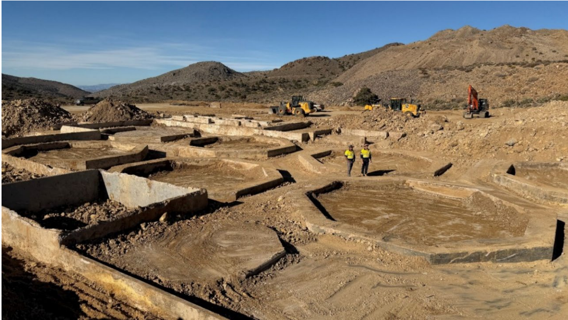
Figure 2: Uncovered concrete structures at Colosseum 5
