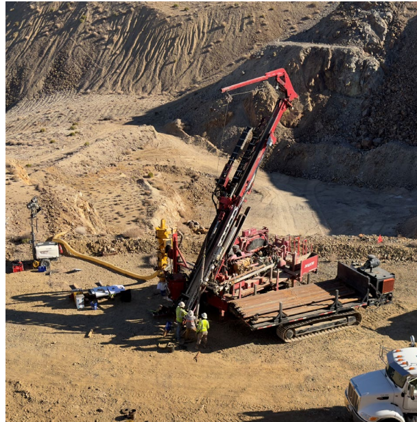
Extensions of pipes at depth
