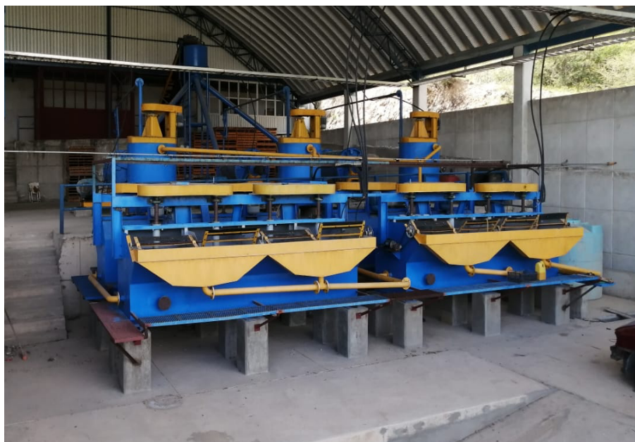
Figure 1. Flotation Cell Banks at Tecmatlán
