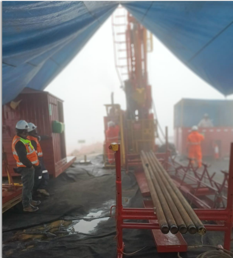
Figure 5. Drill Rig at Parag 25 th January 2024
