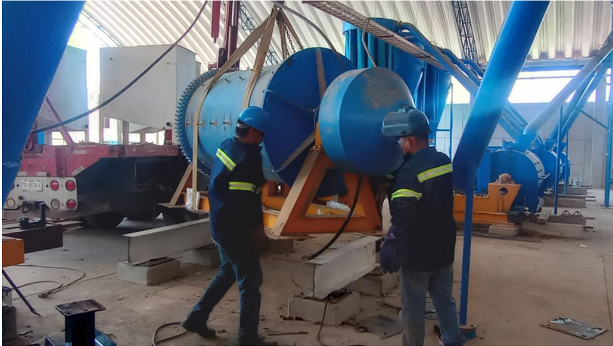
Figure 2 – Mounting of Ball Mill #1.
