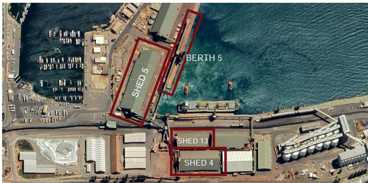
Fenix's Geraldton Port facilities
