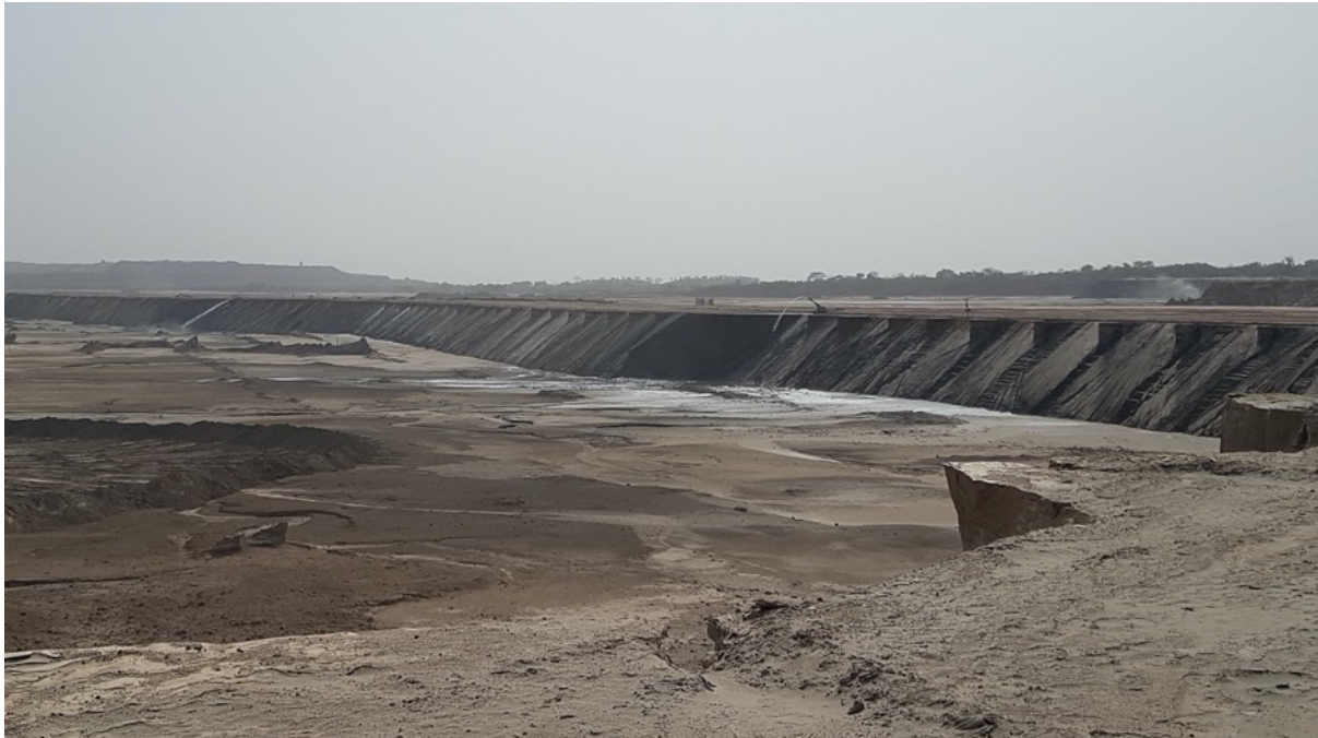
Figure 17: Morila Tailings Storage Facility showing hydraulic mining of upper layer of tailings to expose lower 'higher-grade' tailings
