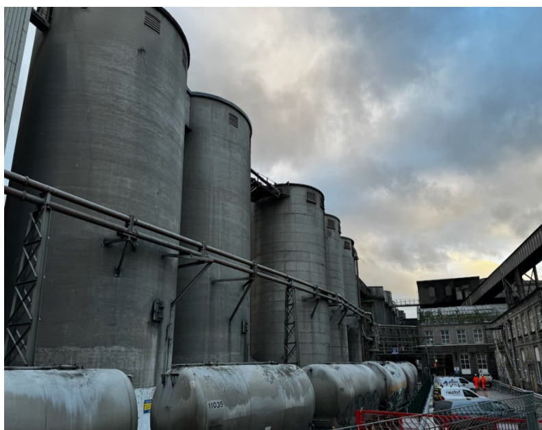
Figures 1-2: (L) Silos at Hope Cement Works containing graphene-enhanced cement. (R) Tiles coming down the production line.
