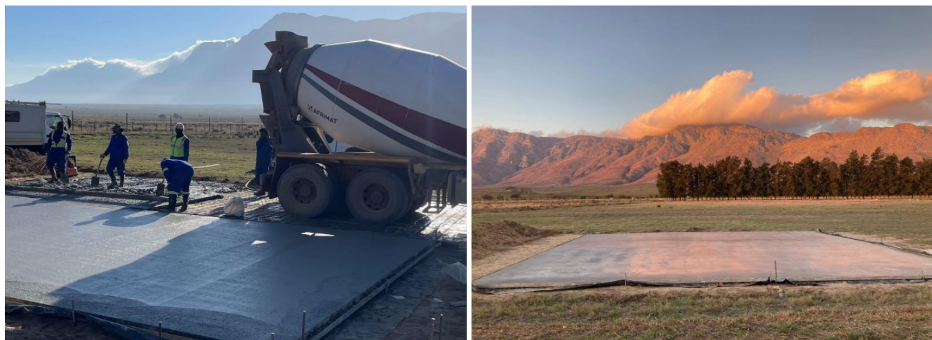
Figure 1: Pouring of the slab at Bontebok Ridge Reserve in South Africa and the slab undercover during curing.
