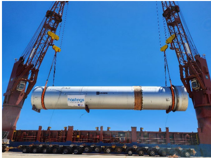
Acid Bake Kiln (weight 100 tonnes)
