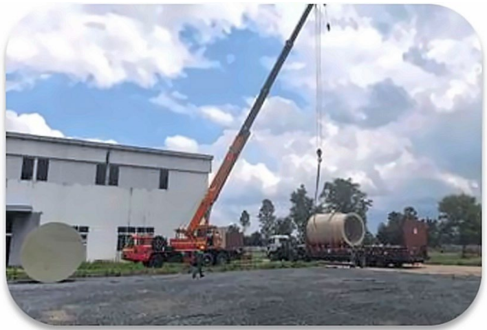
Figure 2 Unloading and handling of process vessel
