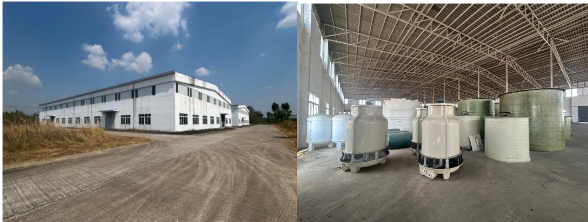
Figures 1 & 2: The Thai Plant facility in Kabin Buri. Executive Chairman Charles Lew, CEO Vince Catania and Head of Business Development Niels Hachmann inspected the Thai Plant in February 2026.
