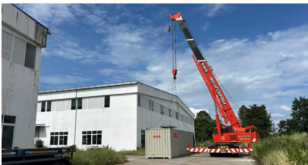
Figure 2: Delivery of plant equipment to site
