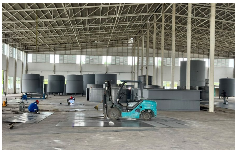
Figure 3: Tank welding and fabrication as part of the upgrade works
