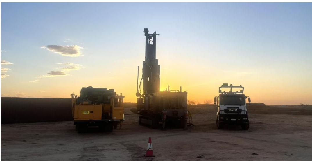
Figure 1: RC Drilling commences at Pippingarra Quarry Project
