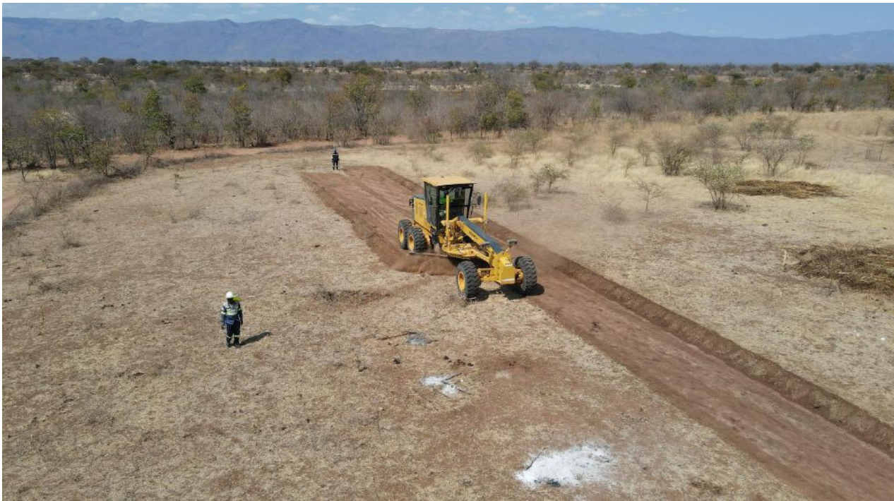
Figure 4 - Musuma-1 Wellpad ground breaking
