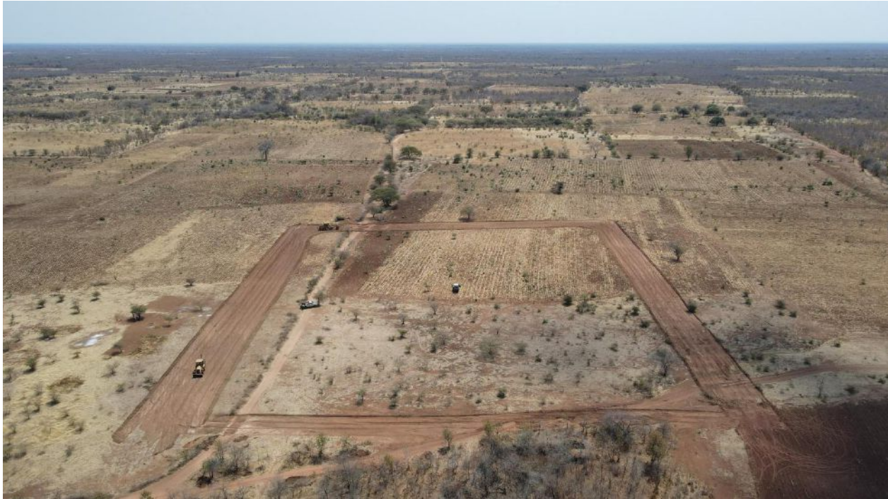
Figure 3 - Musuma-1 wellpad preparation
