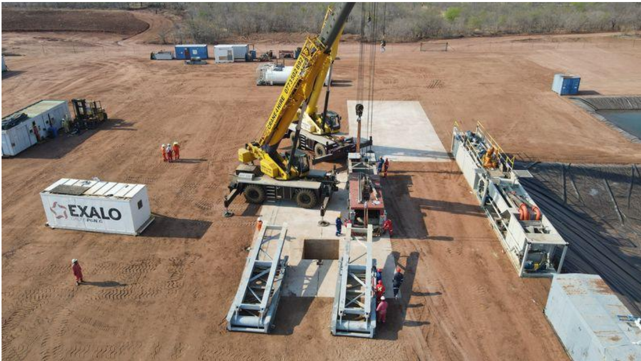
Figure 3 – Rig 202 substructure installation preparation
