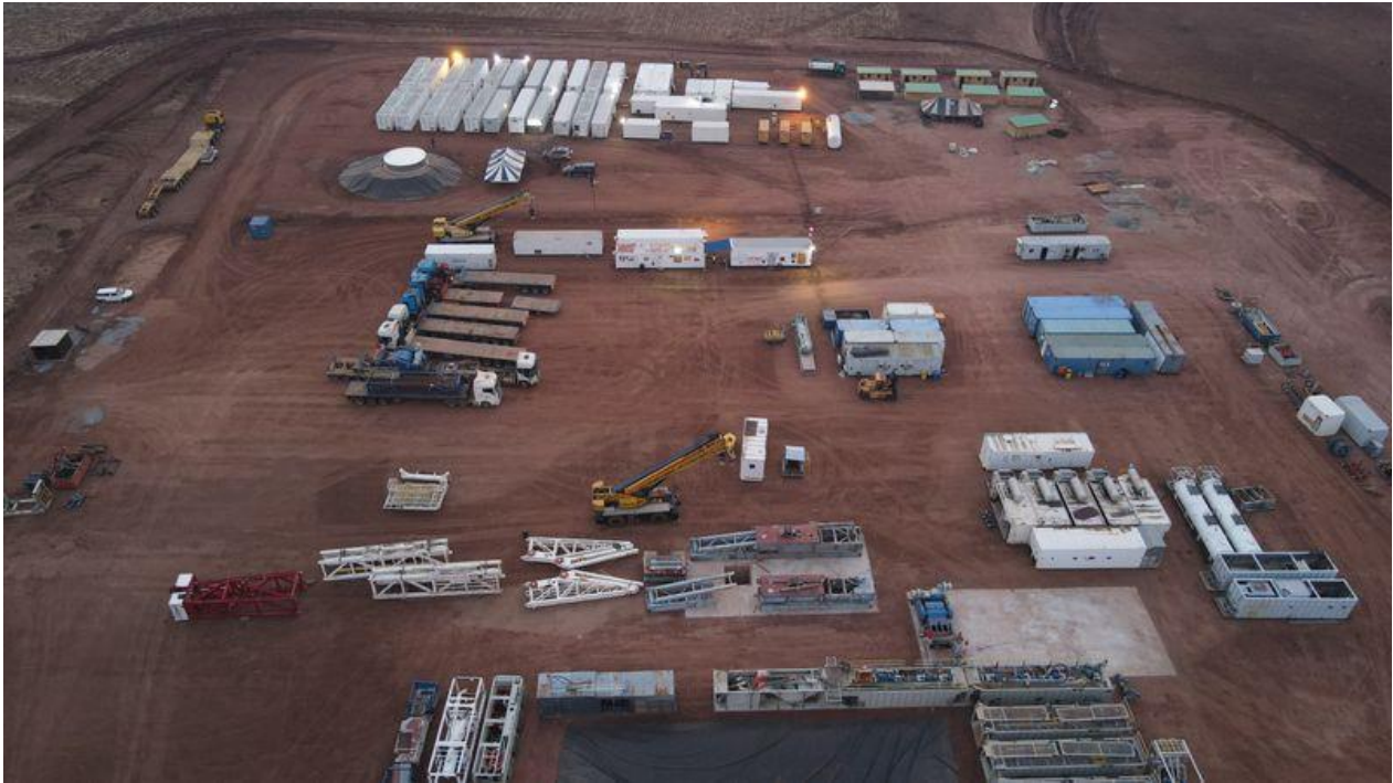
Figure 2 - Musuma-1 wellsite and rig camp aerial view
