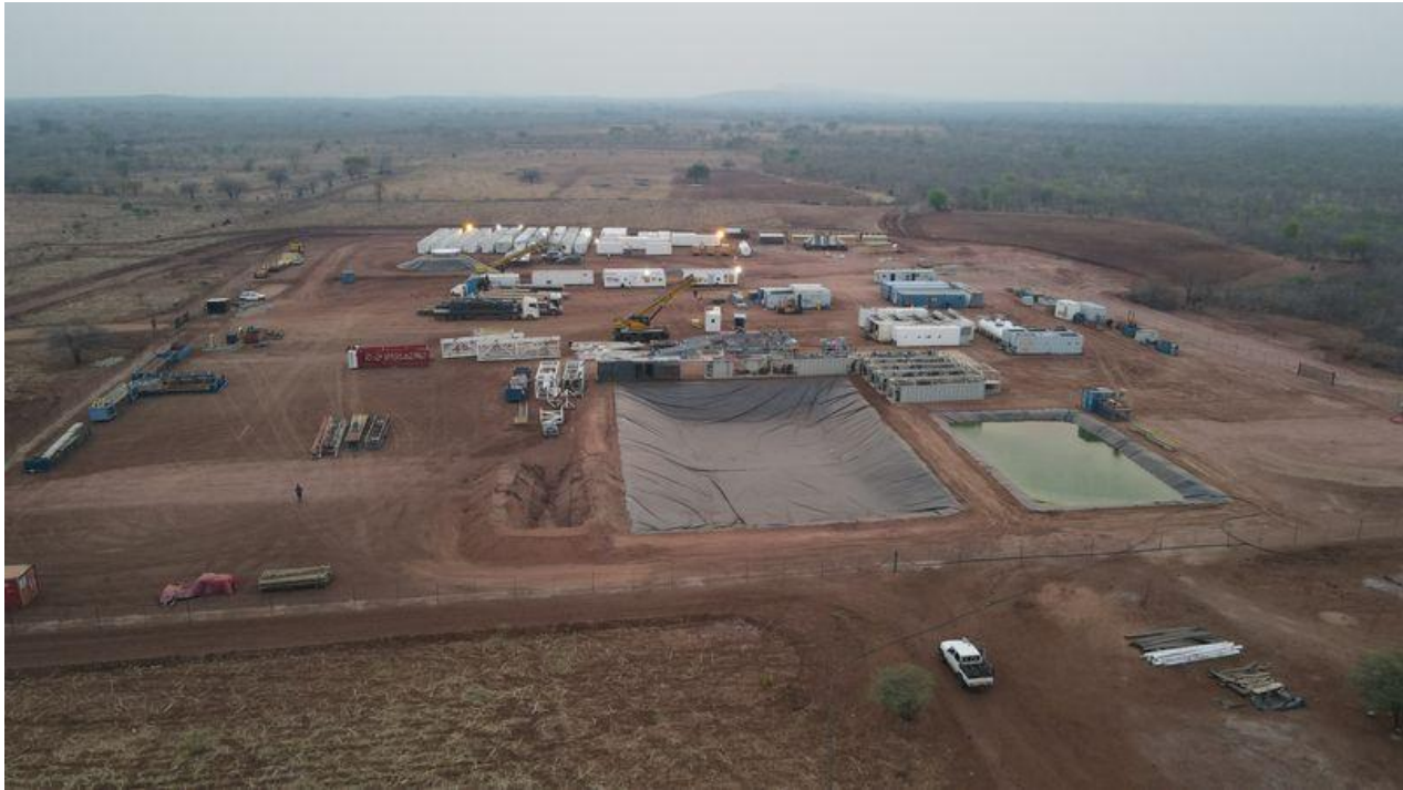
Figure 4 - Musuma-1 wellsite aerial view
