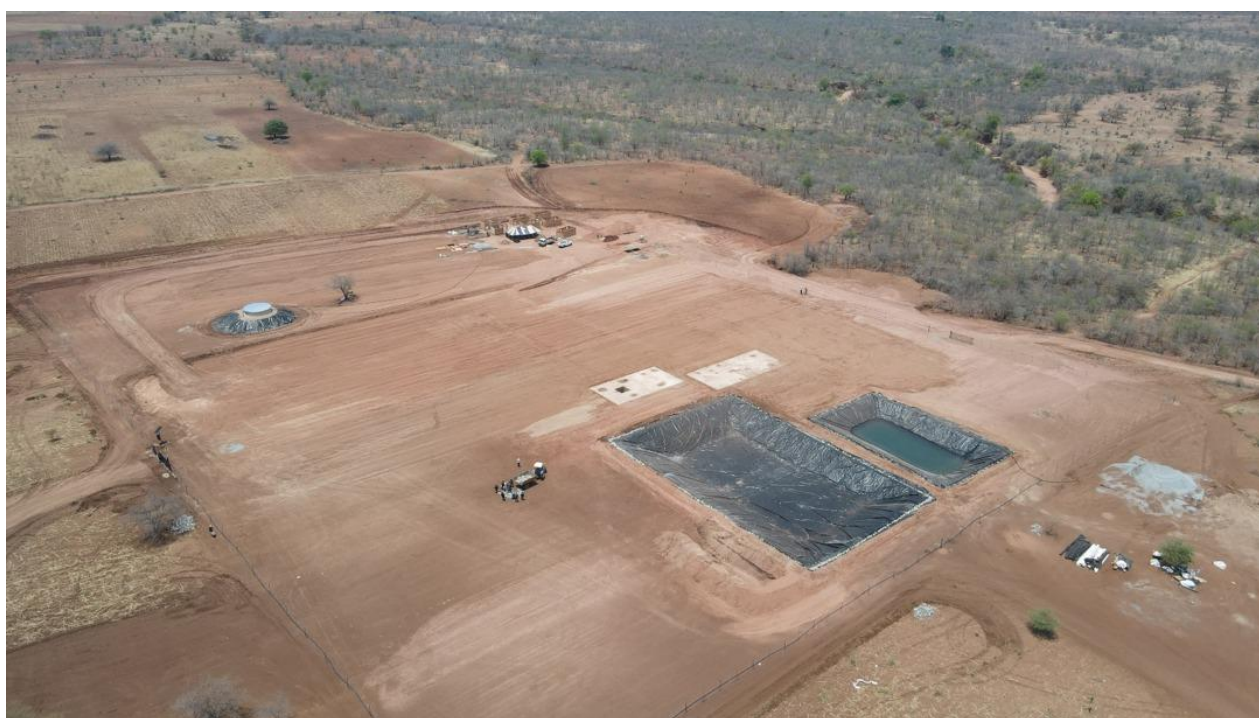
Figure 2 – Completed Musuma-1 wellpad, civil works and access roads, accepted by Exalo in October 2026.
