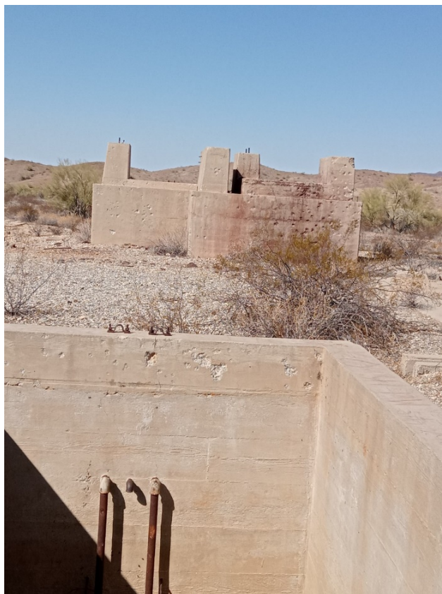
Figure 14 – View of old plant foundations
