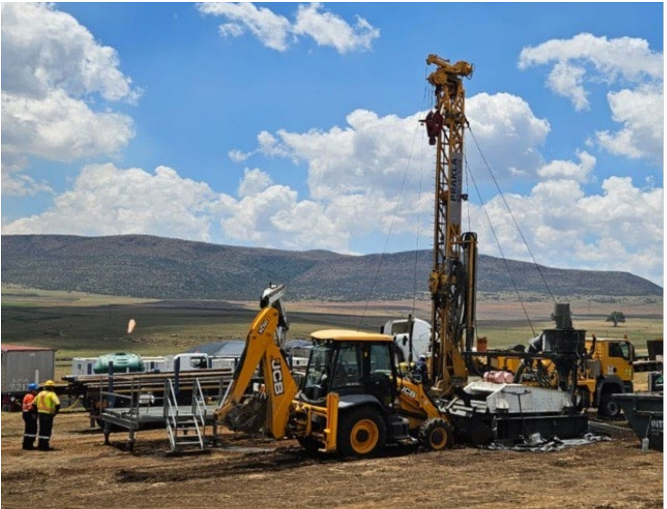
Figure 2 shows the production drilling rig on site for spudding well 271-KV06PT
