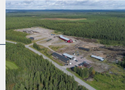
Existing KSB Project office and laydown area
