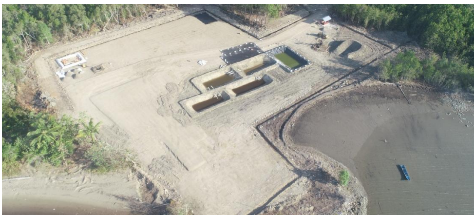
Figure 1: Bula Karang wellsite, ahead of drilling
