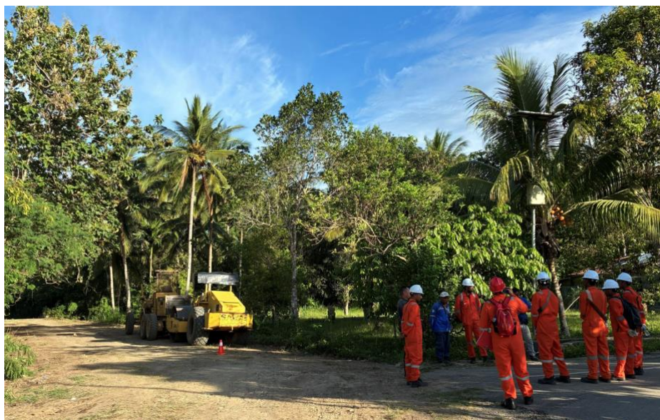
Figure 1: Road access clearing operations
