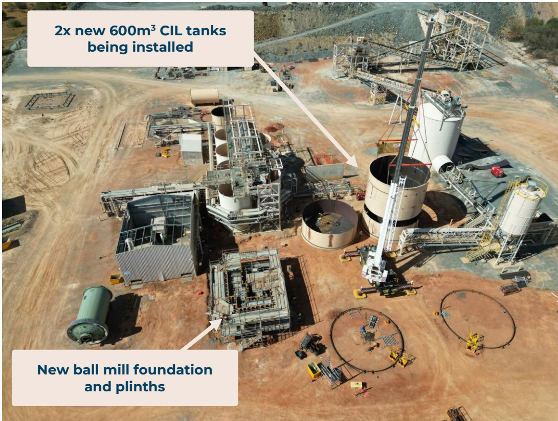
Figure 4: The new ball mill foundation, plinths and tank installation, December 2024.
