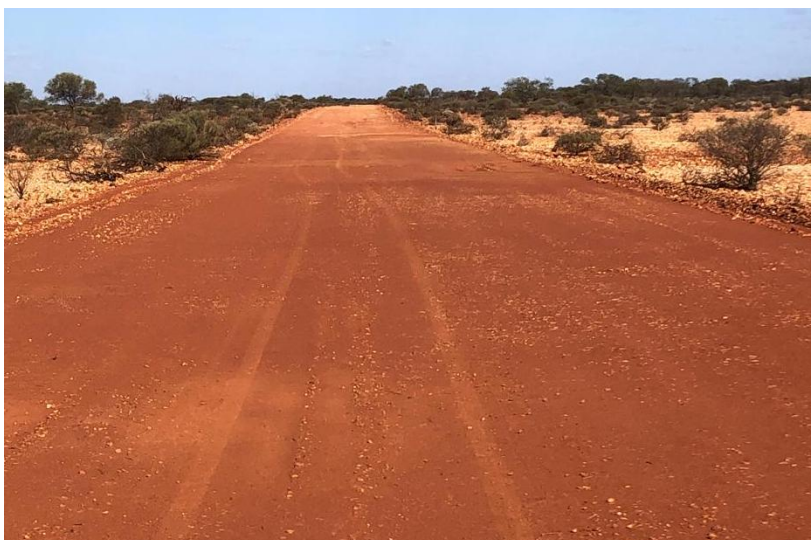
Figure 7: New 20km haul road, November 2024.
