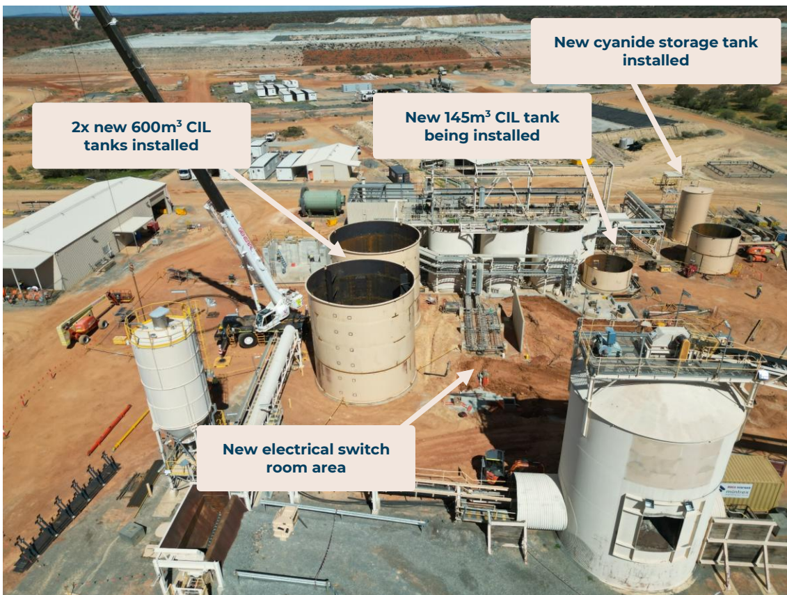
Figure 4: Progress on the expanded processing plant, January 2025.
