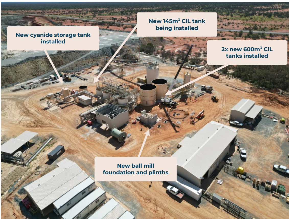
Figure 3: Progress on the expanded processing plant, January 2025.
