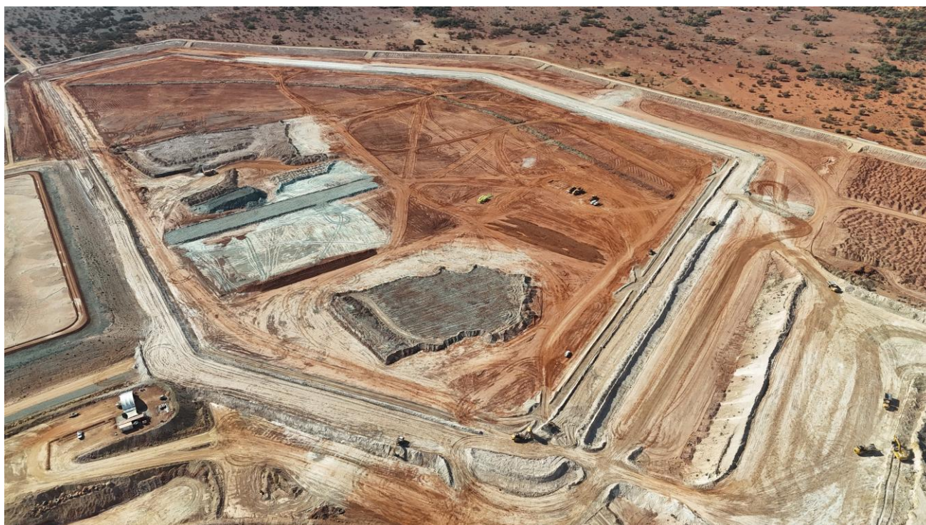
Figure 7: Stage 1 of the new TSF under construction.
