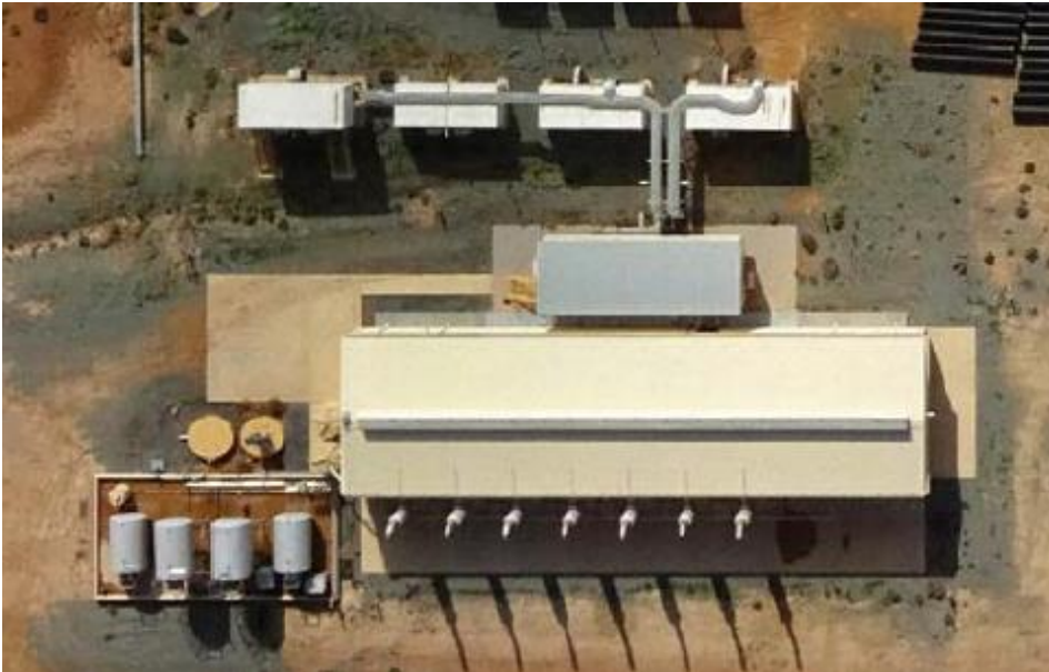
Figure 52 – Andy Well power station.
