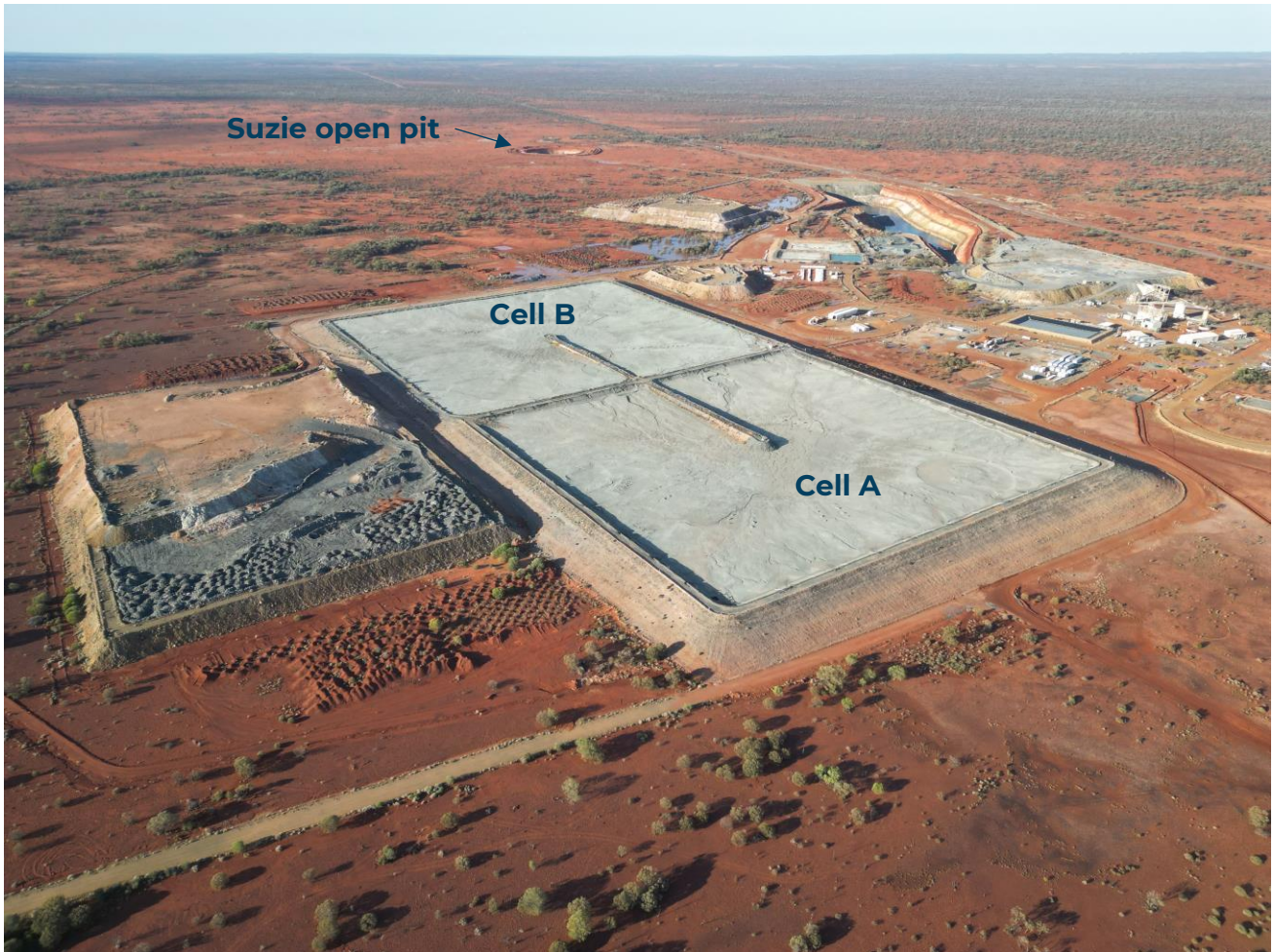
Figure 42 – Existing TSF, December 2024.
