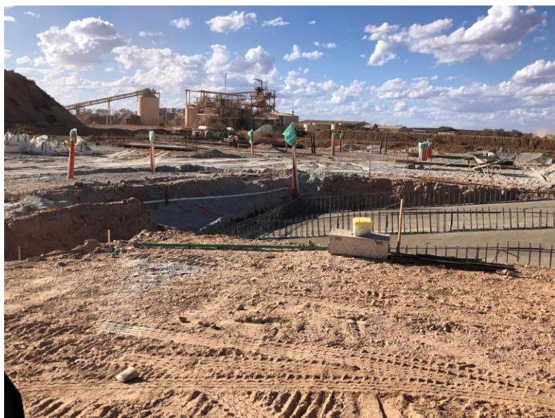
Figure 5: Wash plant pad and sumps.
