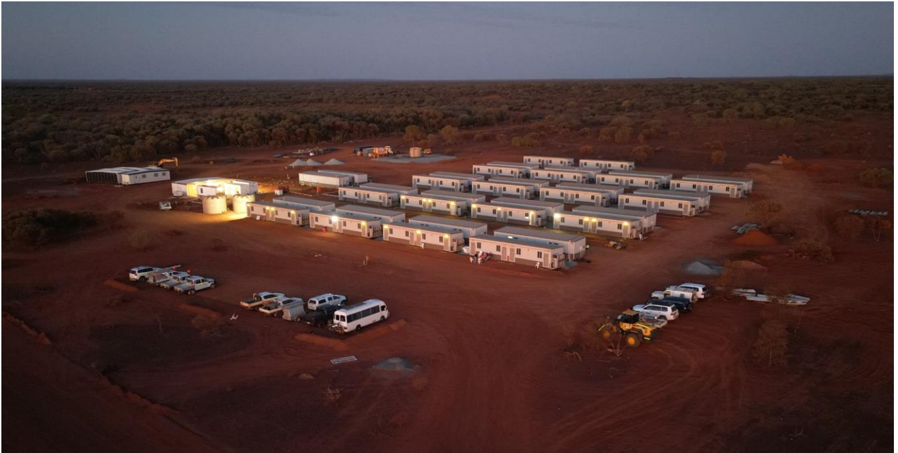
Figure 1: 136-person accommodation village, October 2024.
