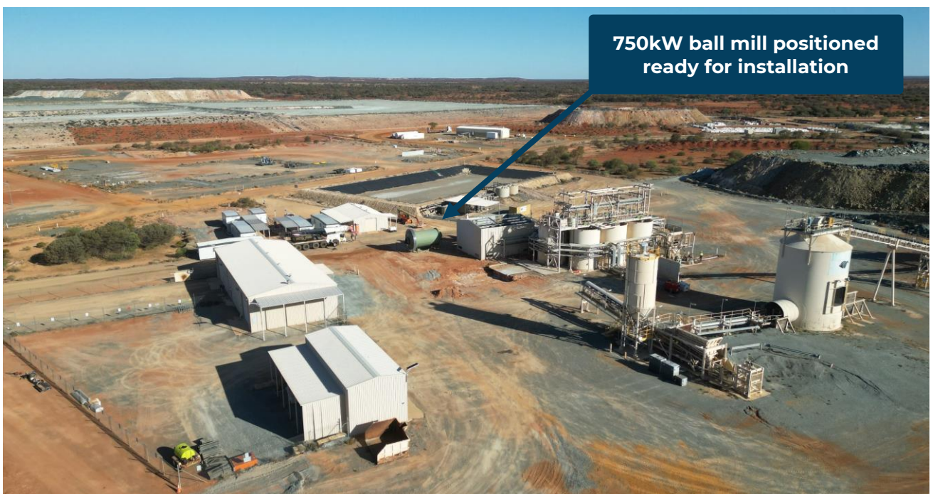
Figure 4: 750kW ball mill unloaded and ready for installation at the Murchison.
