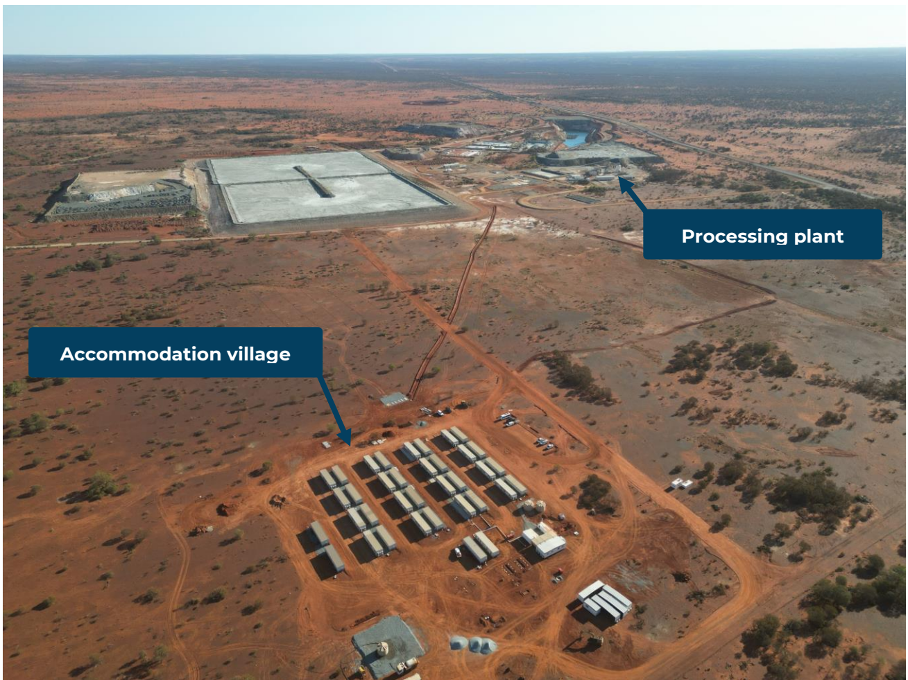
Figure 2: 136-person accommodation village relative to other infrastructure, October 2024.
