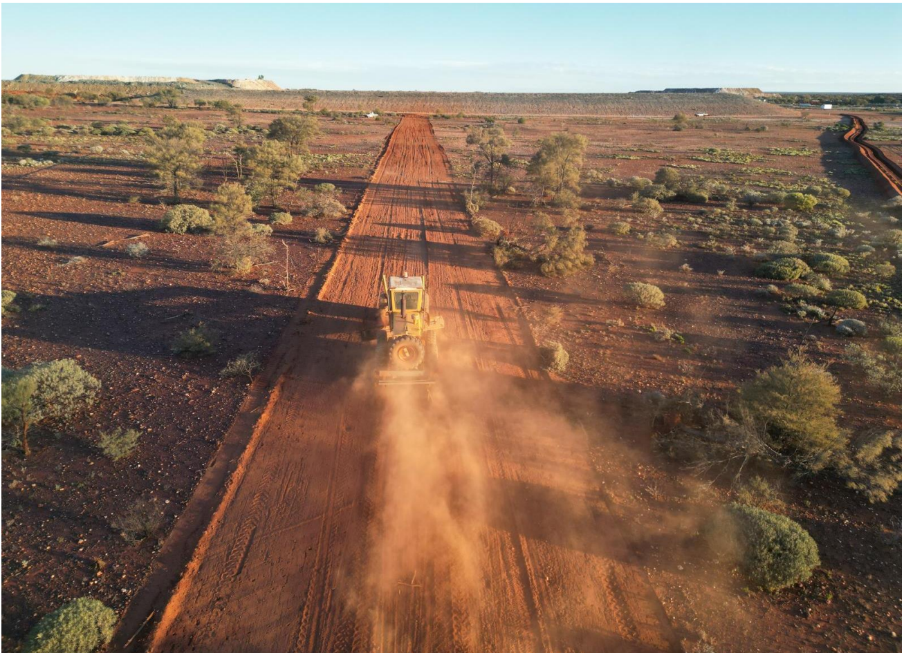
Figure 1: Haul road construction underway, July 2024.
