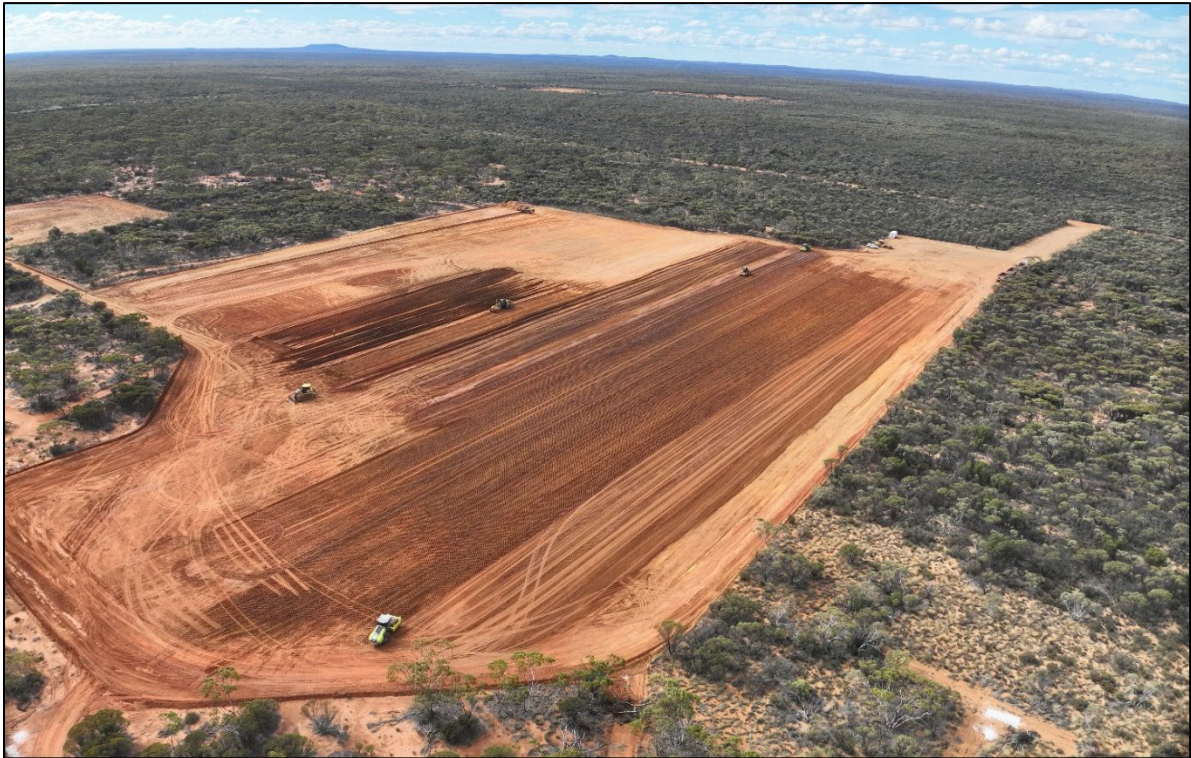
Figure 1: Village site preparation and bulk earthworks
