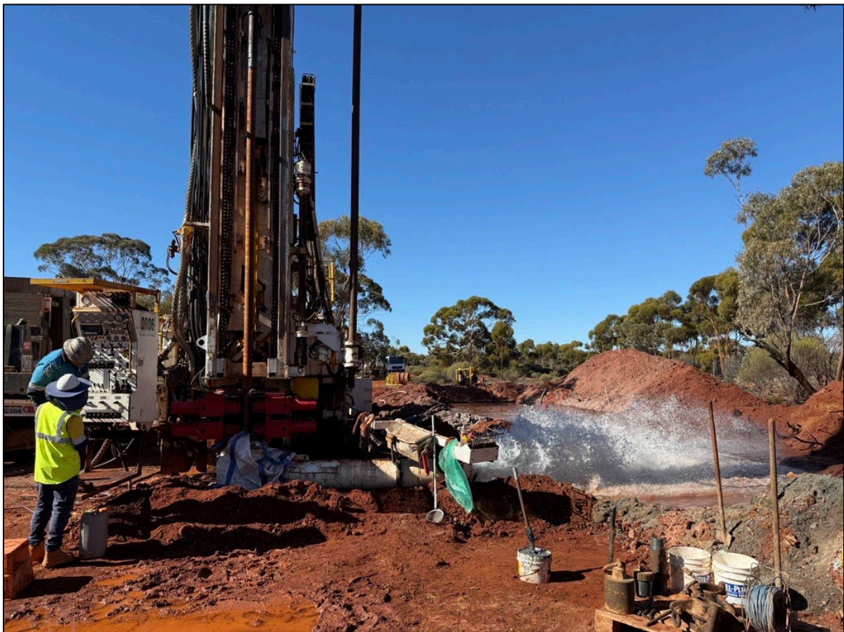
Figure 2: Water bore airlift testing
