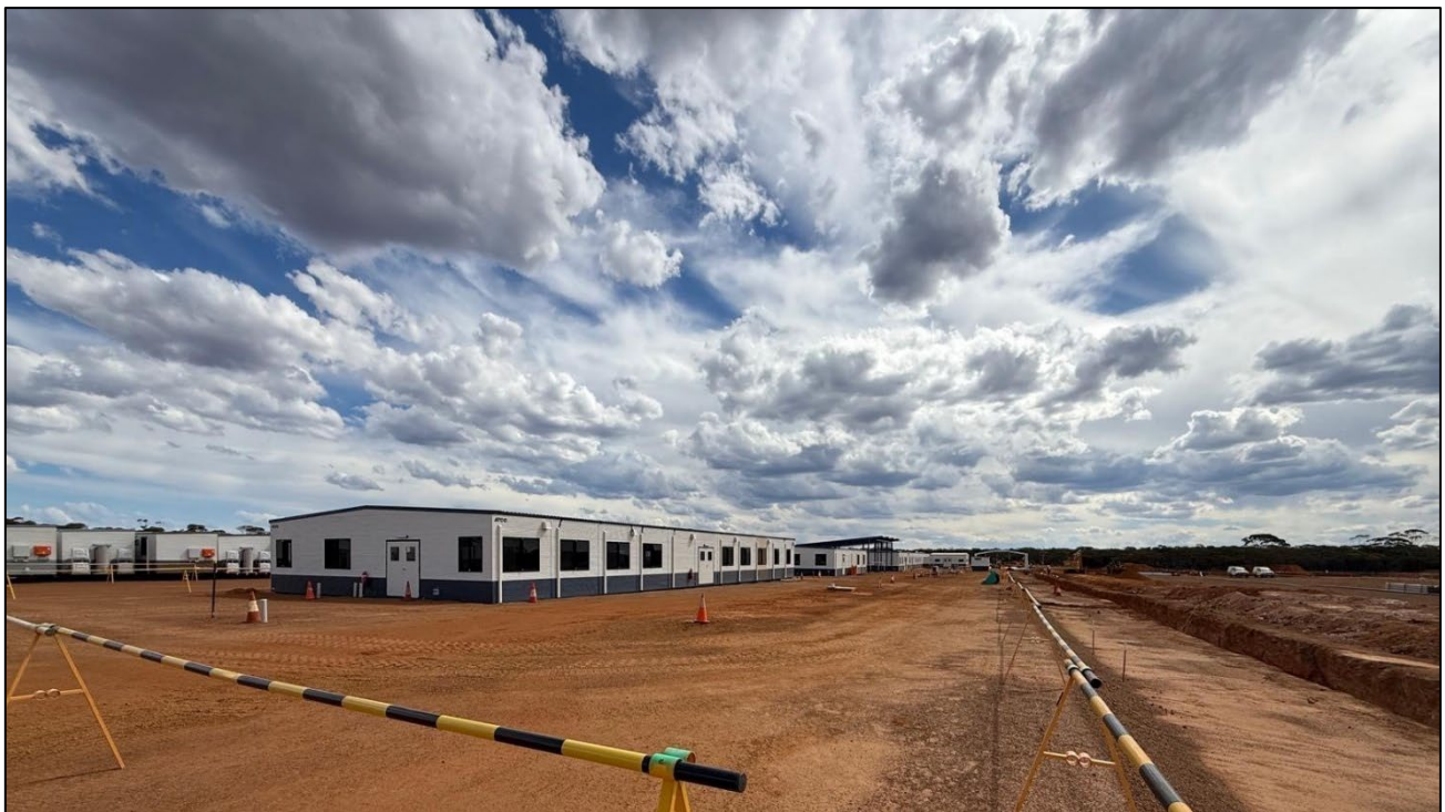
Figure 4: Village construction progress – gymnasium, administration building and social hub
