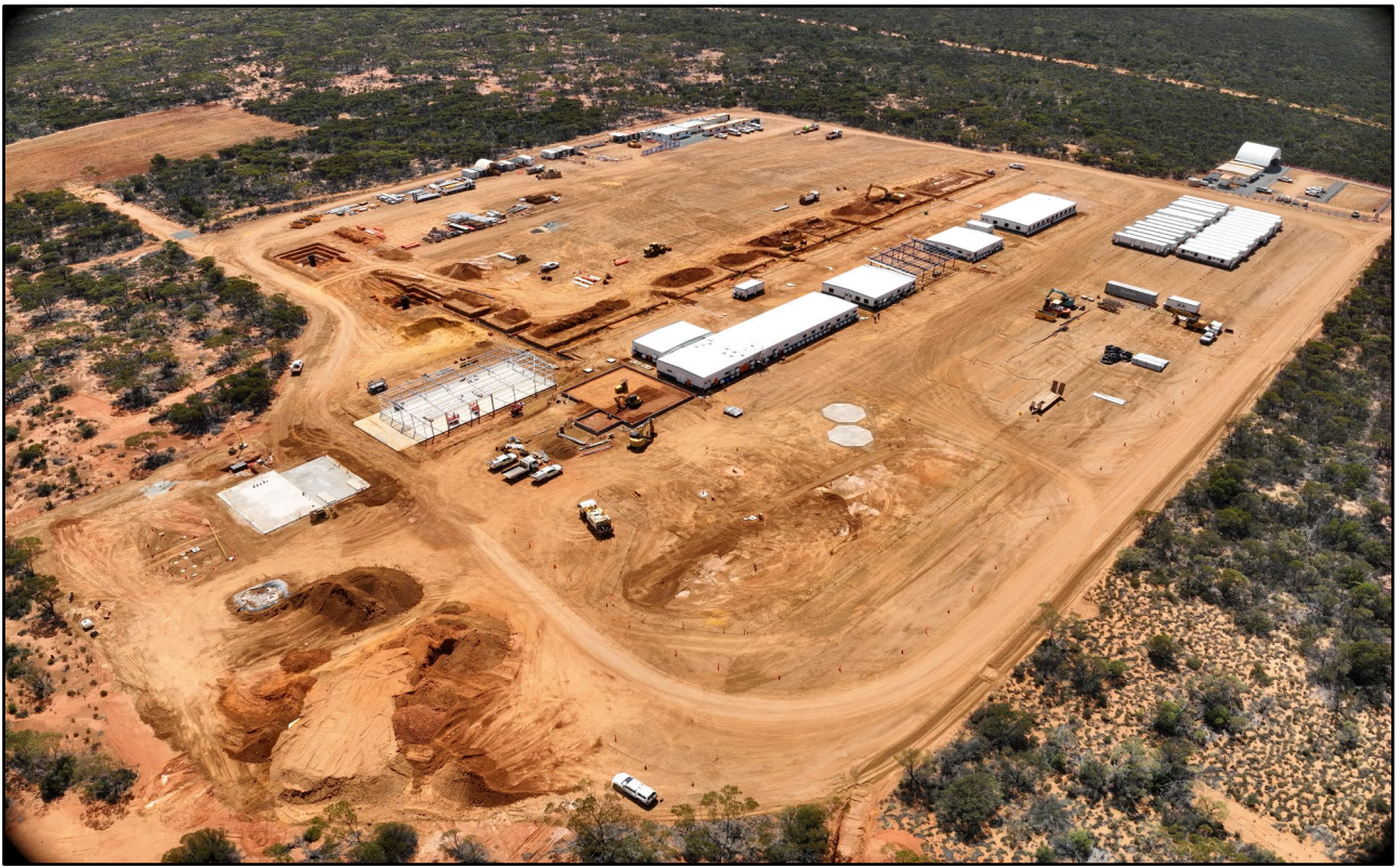
Figure 3: Village construction progress – aerial view
