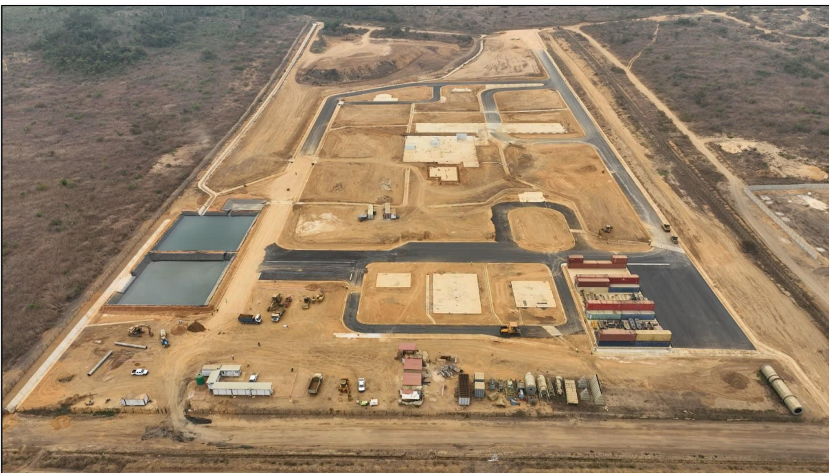
Fig .2. Minor civil works being finalised at Subantando Fertilizer Factory.
