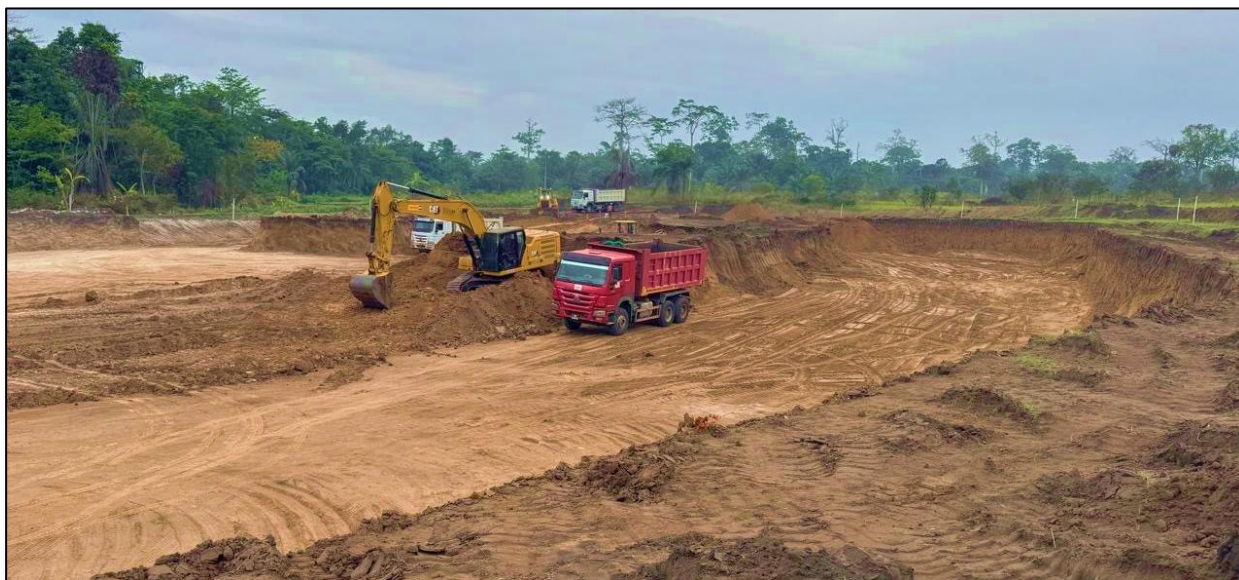
Figure 2: Active excavation and haulage fleet operations opening up initial excavation horizons at Cacata.
