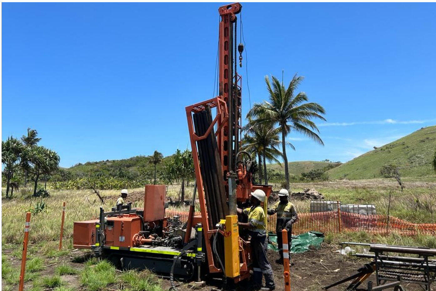
Geotechnical Drill Rig being Setup, October 2023
