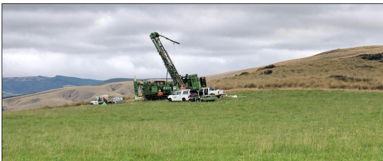
Figure 5 : Photo of drill rig on first target prorc0009 at Lammerlaw
