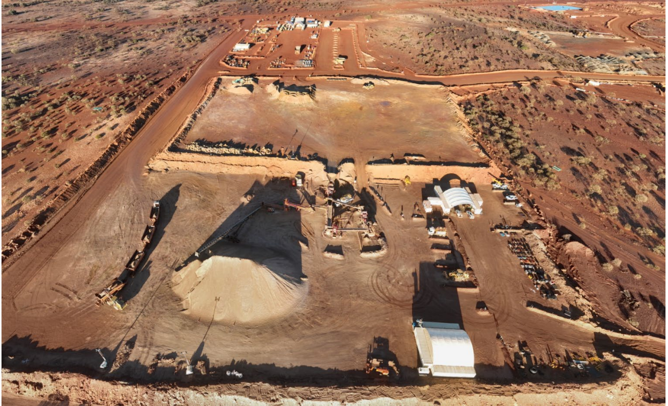
Figure 4: Crown Prince Gold Mine ROM, Crusher and Crushed Ore product stockpile area
