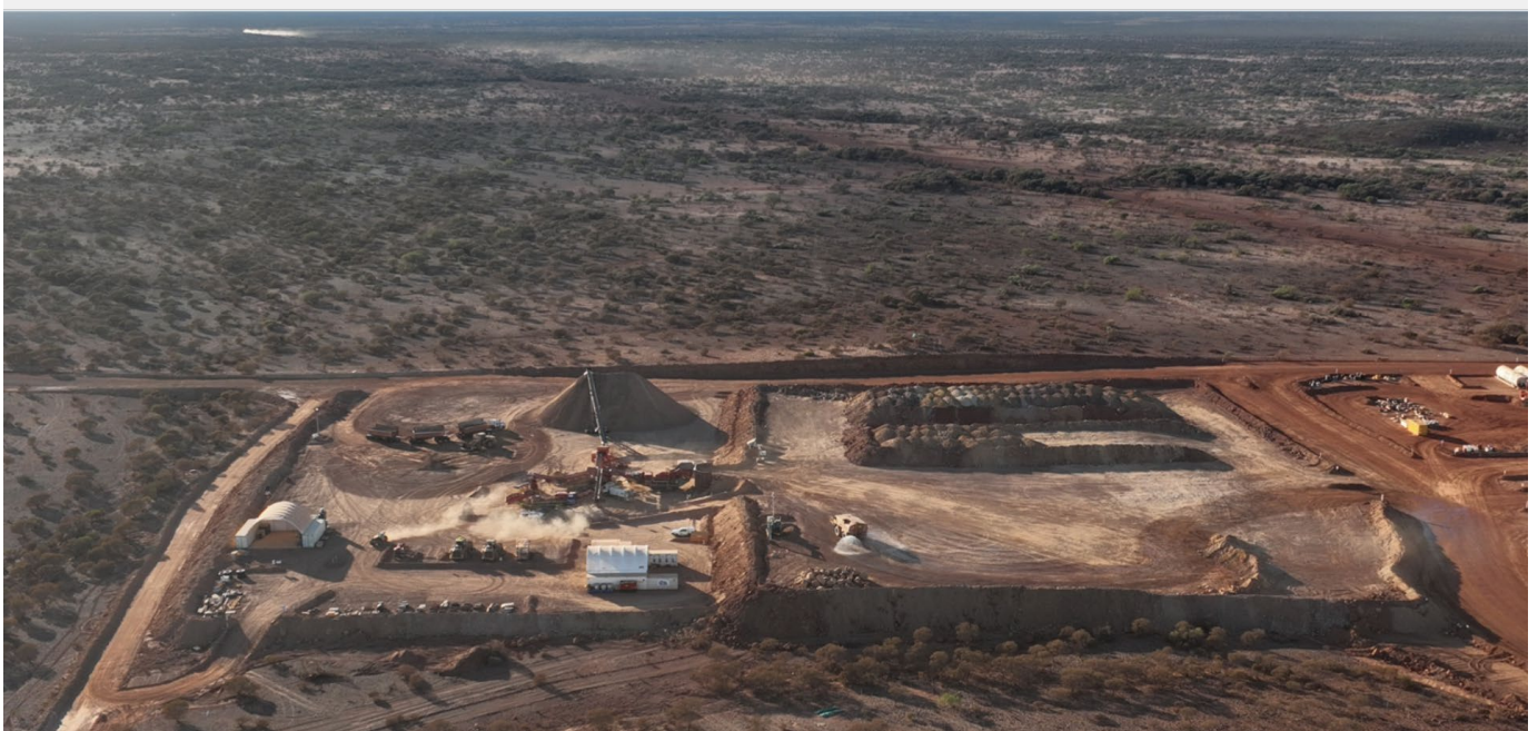
Figure 2: Crown Prince ROM and Crusher Pad
